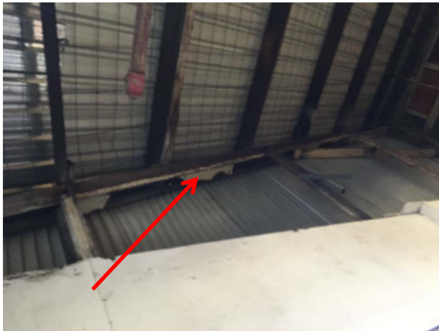
Location: 182-198 Victoria Road & 28-30 Faversham Street, Marrickville, NSW – Stone Cutting Workshop The red arrow points to the asbestos cement sheeting roof partition on the eastern wall
