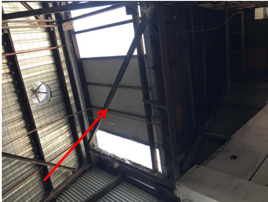
Location: 182-198 Victoria Road & 28-30 Faversham Street, Marrickville, NSW – Stone Cutting Workshop The red arrow points to the asbestos cement sheeting window infills on the southern windows of the eastern wall
